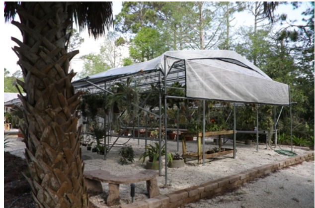
2. The shade structure is covered with 50% shade cloth; a second layer is not required because of the buoyant air movement. Styrofoam fills the bottom half of the pots for improved drainage during tropical storms.
