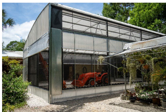
Time for a new greenhouse!
