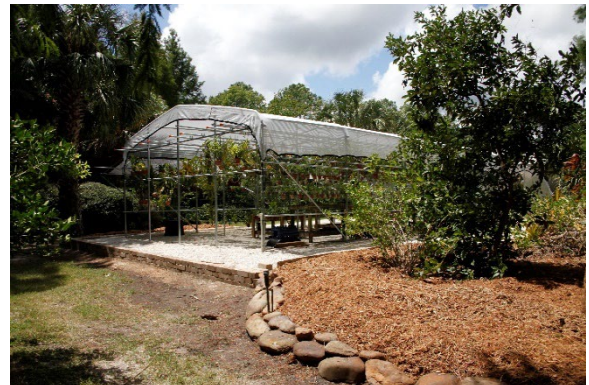
How about a big shade structure to summer orchids outdoors, with lots of air movement?
