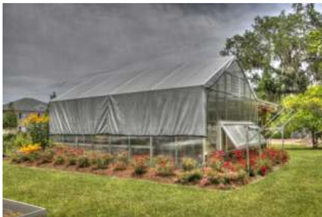
The Atlas greenhouse is a polycarbonate structure covered in 65% shade cloth, complete with water wall for summer cooling and furnace for winter heating.
